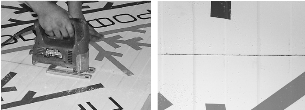
Figure 10. Cutting of the panel with the jigsaw and the resulting cutting line.
