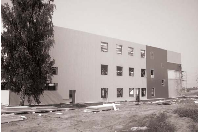
Figure 67. Sandwich panel building with the vertical placement (Moscow region, Reutov town).
