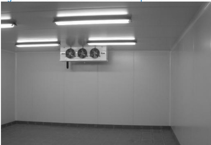
Figure 25. Room made with sandwich panels
