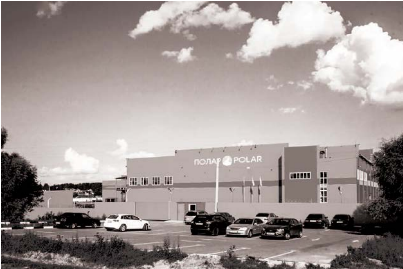
Figure 66. Industrial building with the horizontal panel placement (Moscow region, Shelkovo town).
