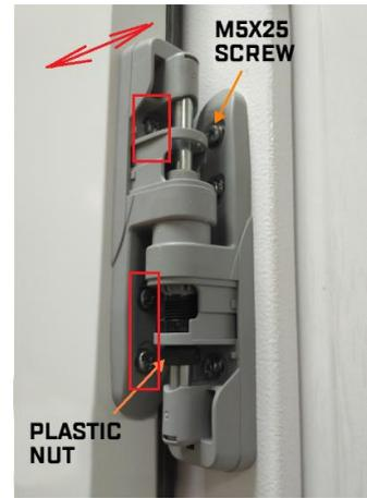
Adjusting the position of the leaf relative to the opening should be carried out in the following order:
